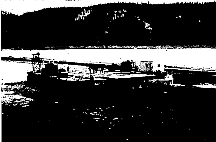
Hoverbarges were winched across with cables.
